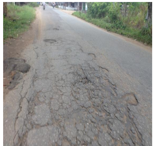
Foto 1: Alligator cracking or Map cracking (Fatigue)- Kabupaten Kubu Raya
